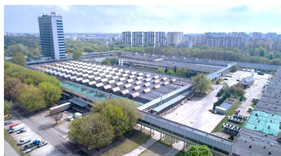
Photo: CeMat complex, Wólczyńska 133, Warsaw, Poland
