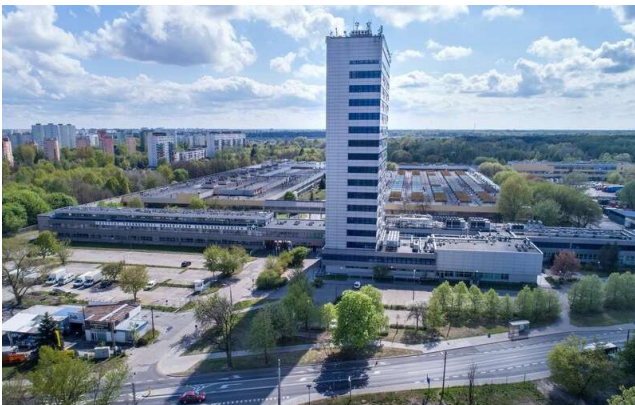
CeMat & PKO BP office building
